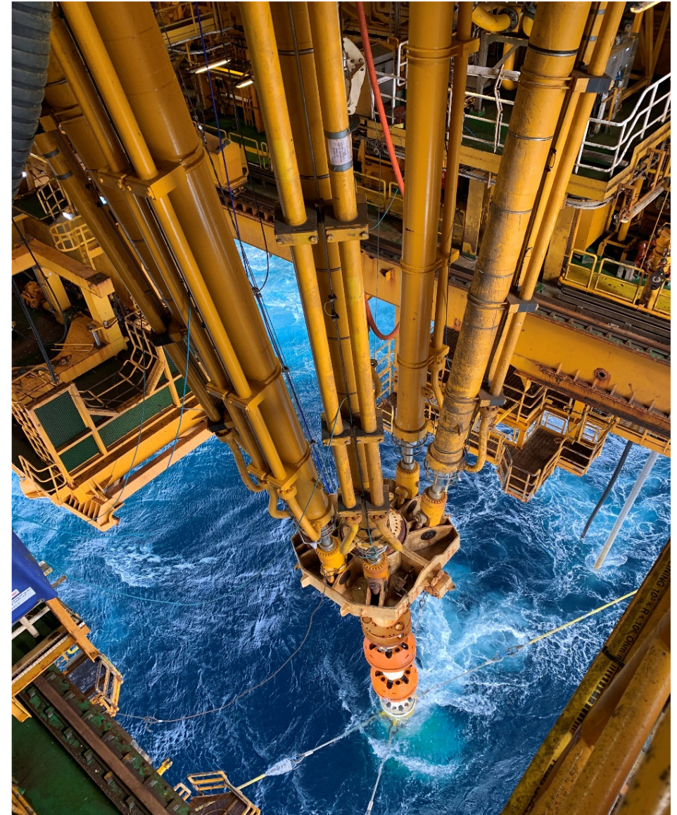
The Odfjell Deepsea Stavanger rig will drill the Luiperd Prospect on Block 11B/12B offshore South Africa.
